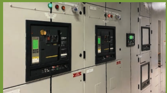
Electrical Panel Upgrades
