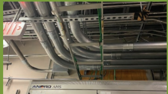
Electrical Wiring Modernization
